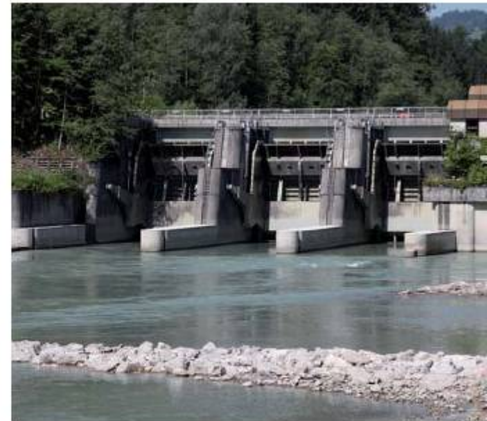
■ Figure 8.15 Hydroelectric power plant
