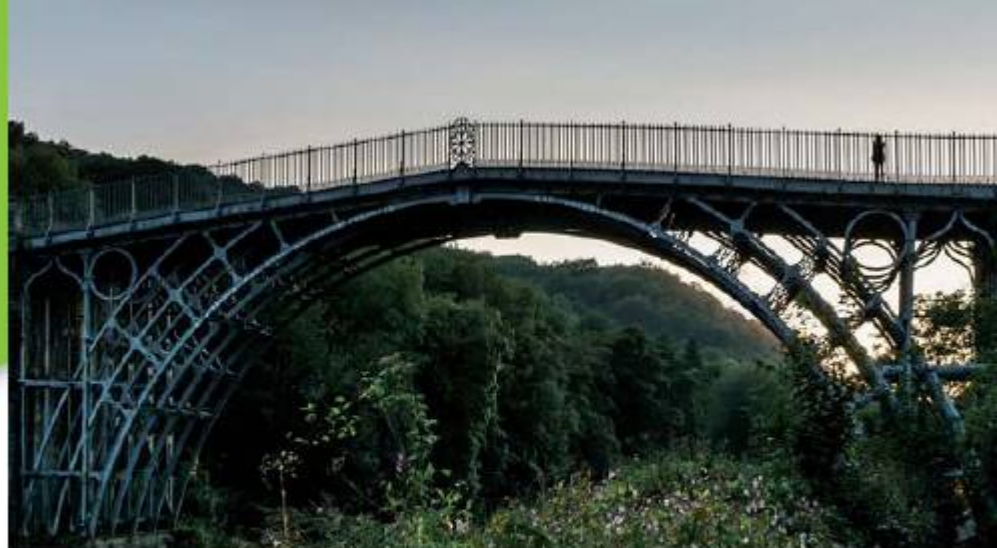
■ Figure 3.34 The Iron Bridge, Shropshire, UK
