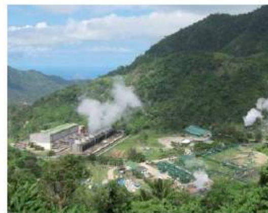
■ Figure 8.21 Geothermal power station
