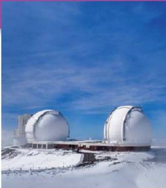
■ Figure 12.17 The Keck telescopes at Mauna Kea observatory, Hawaii, use 10m diameter mirrors with 17.5m focal lengths
