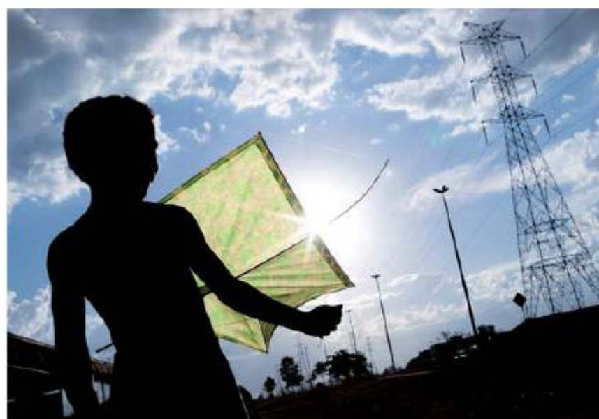
■ Figure 9.29 Flying kites under high voltage cables is very dangerous indeed
